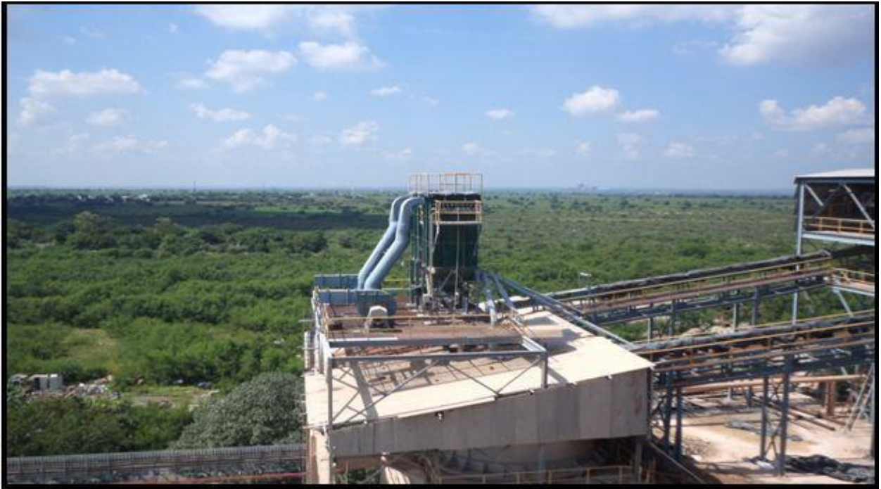
Tree Plantation inside the factory premises
