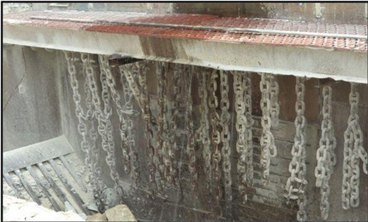
Water spray system installed in crusher
