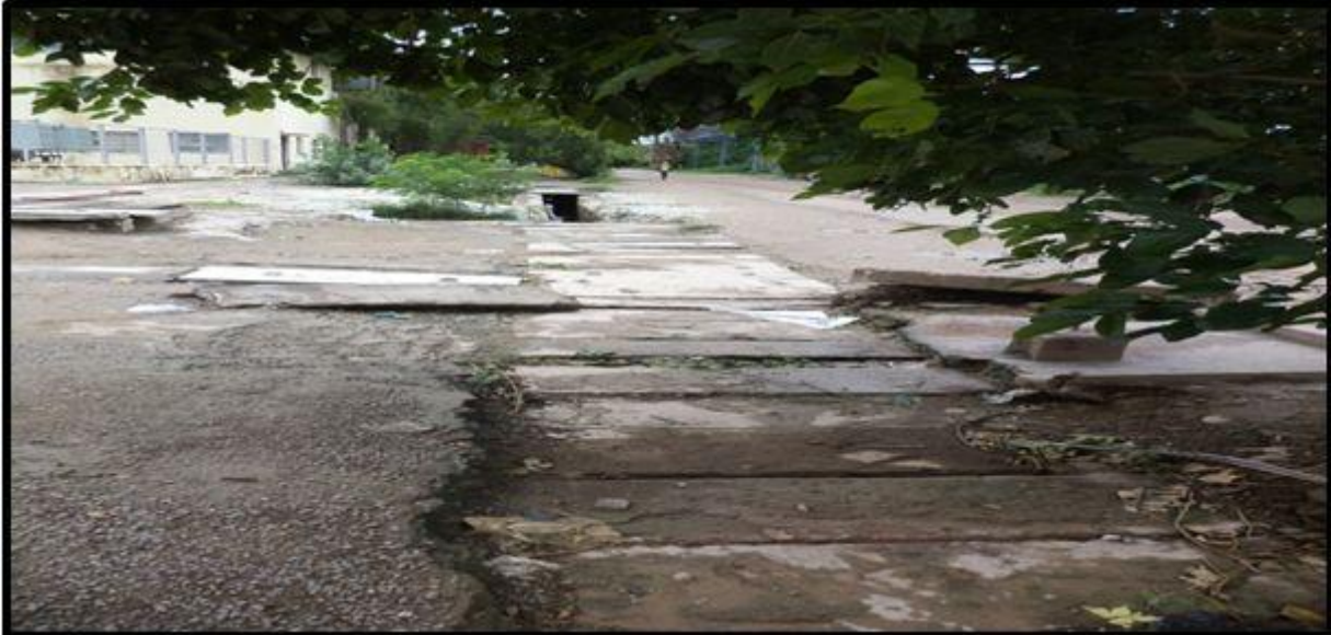
Storm Drains leading to Mines pit
