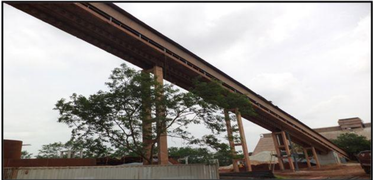
Covered belt conveyors
