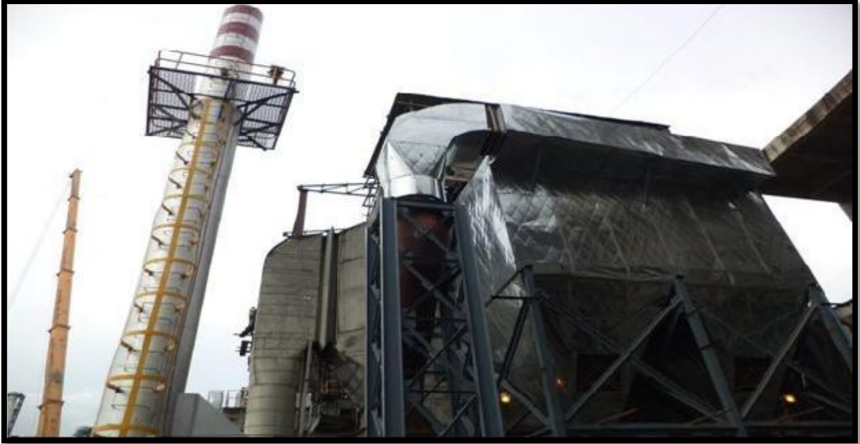
Cement Mill-2 Bag filter
