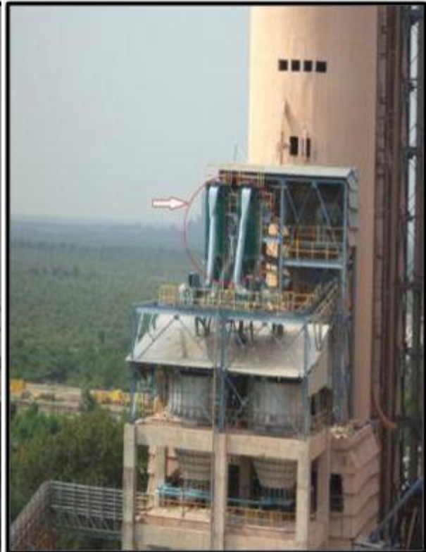
Bag Filter Installed in kiln feed section
