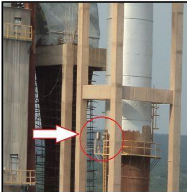
Continuous Emission monitoring Analyzer on Coal mill stack
