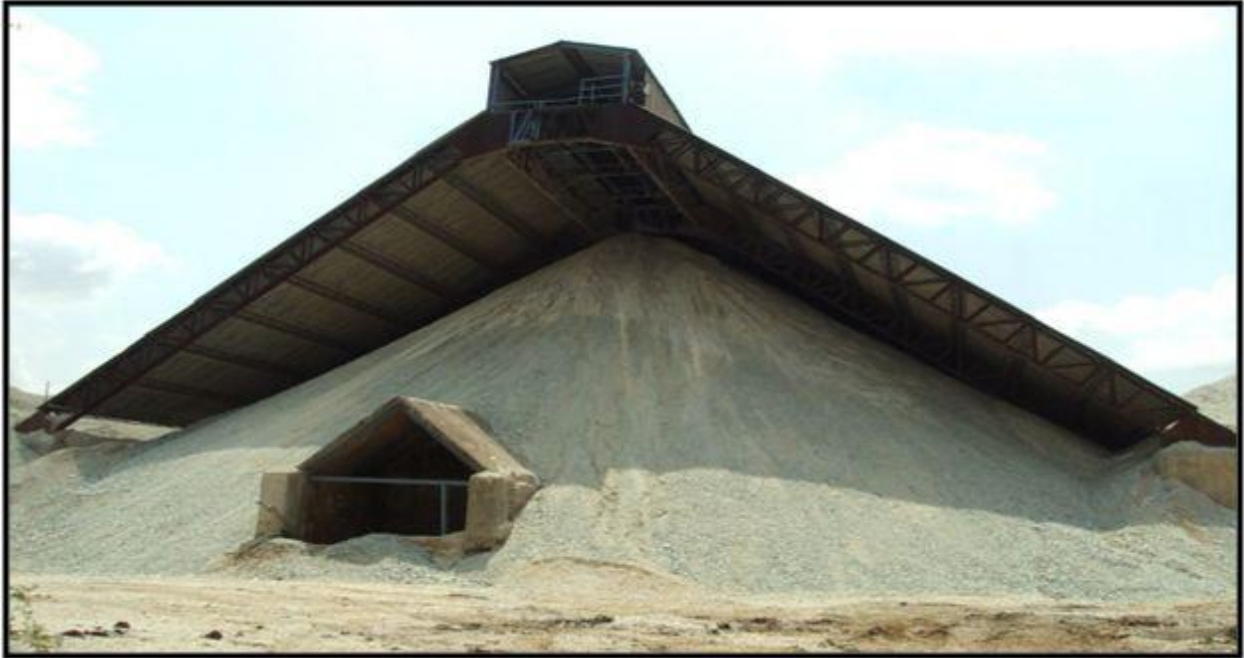
Crushed lime stone yard
