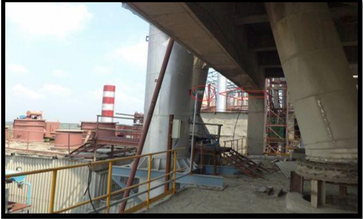
Continuous Emission monitoring Analyzer on Cement mill-1
