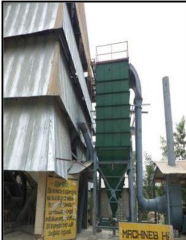
Bag Filter Installed on Crusher
