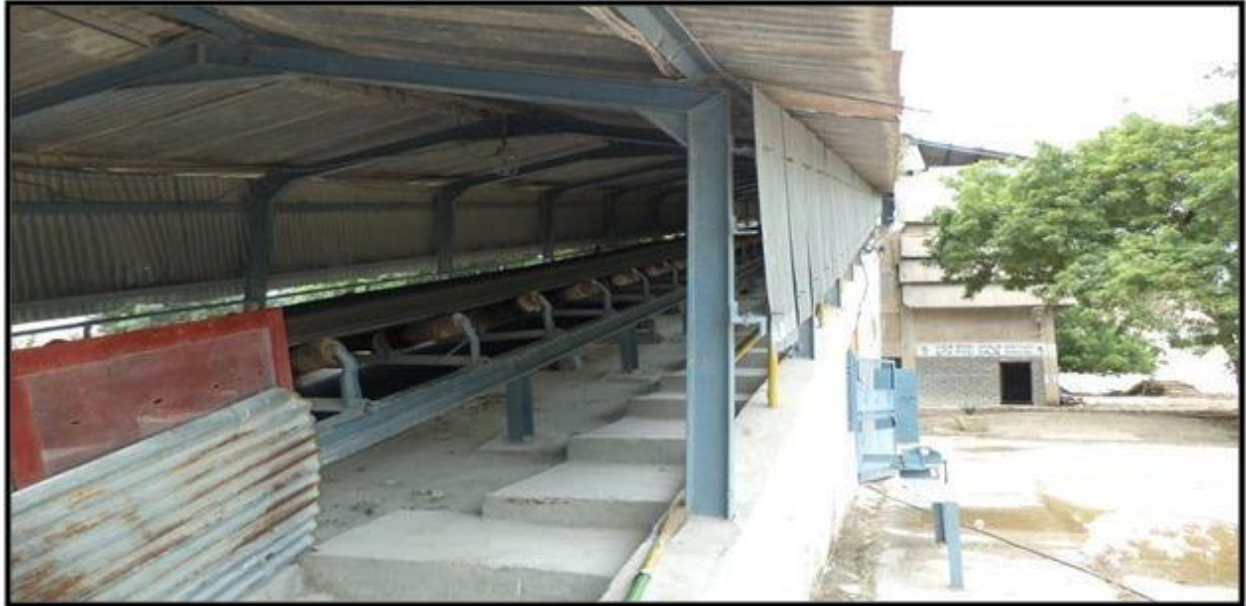
Covered belt conveyors
