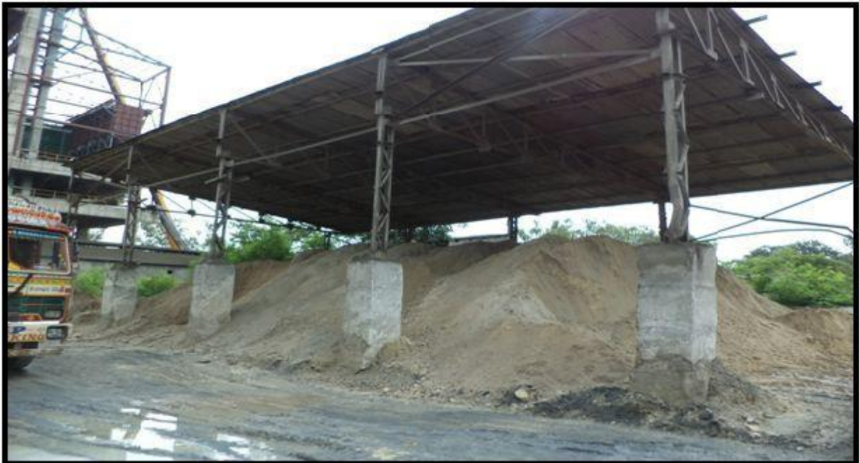
Coverd Gypsum yard
