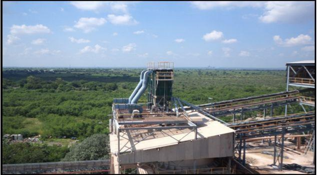
Tree Plantation inside the factory premises
