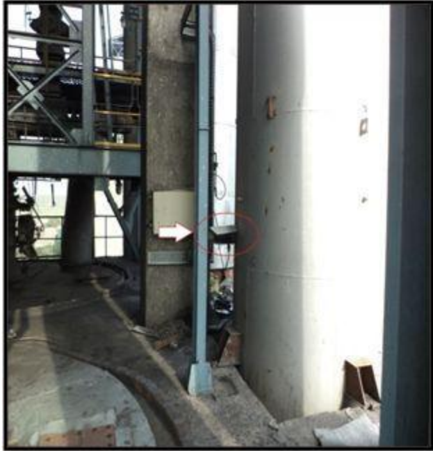
Continuous Emission monitoring Analyzer on Coal mill stack
