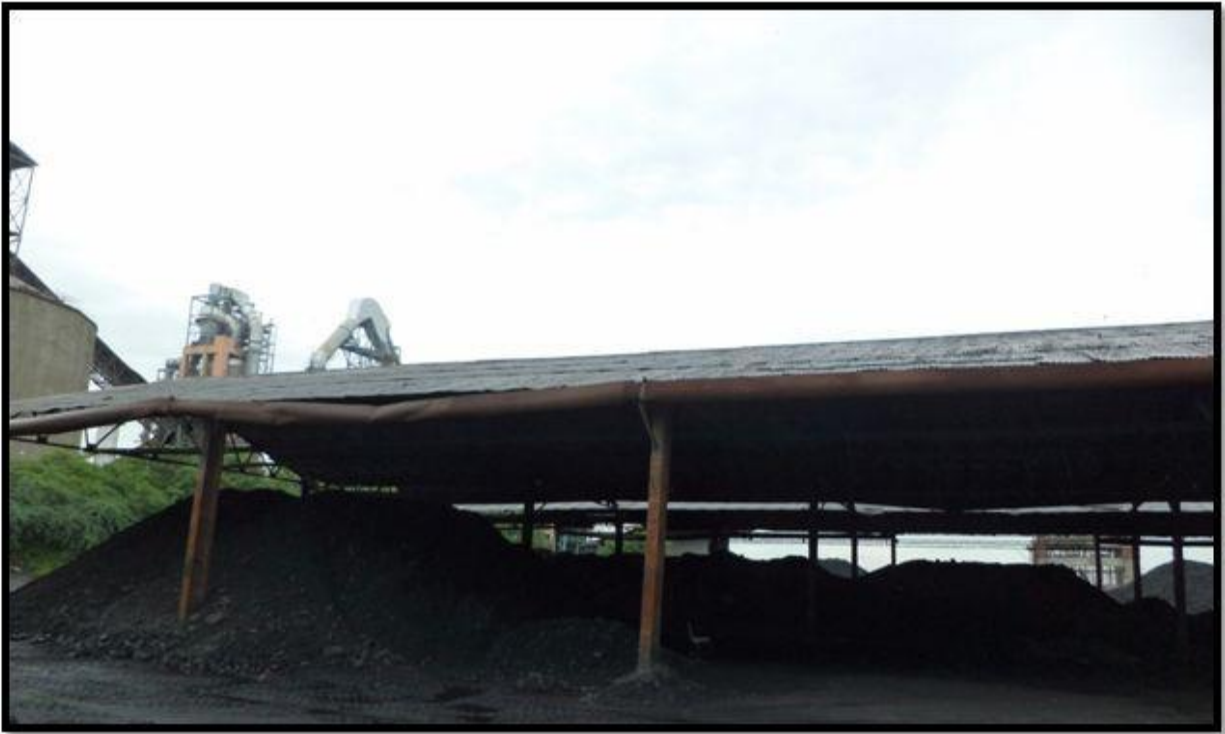
Covered Coal yard
