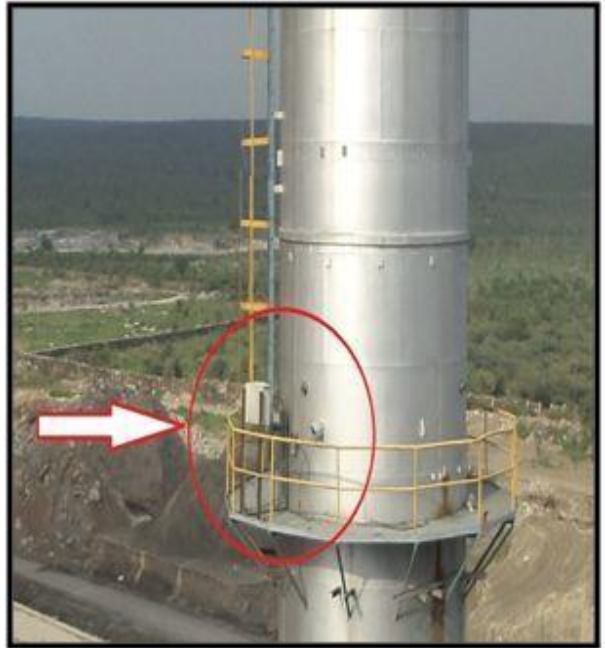
Cooler ESP Stack
